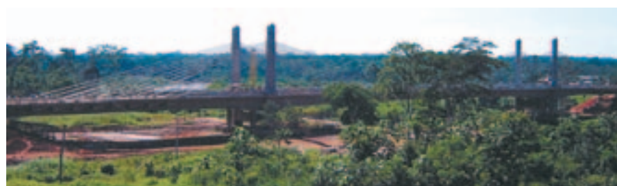
A 20 km-long bridge over the Zaire River will facilitate communication with Cabinda
