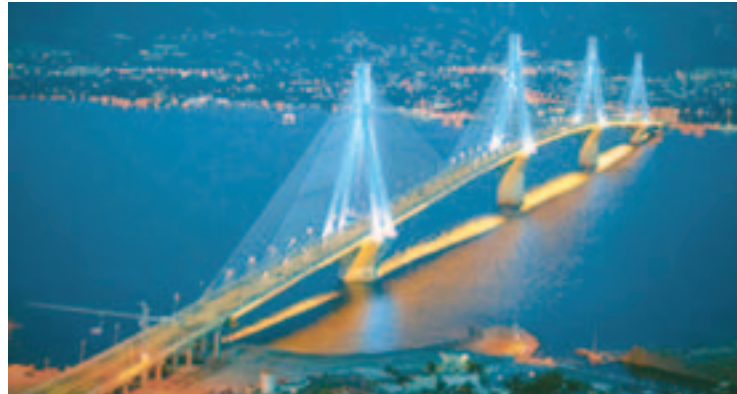
The Rio-Antirio Bridge cost a total of £630 million and was funded by the EU.
