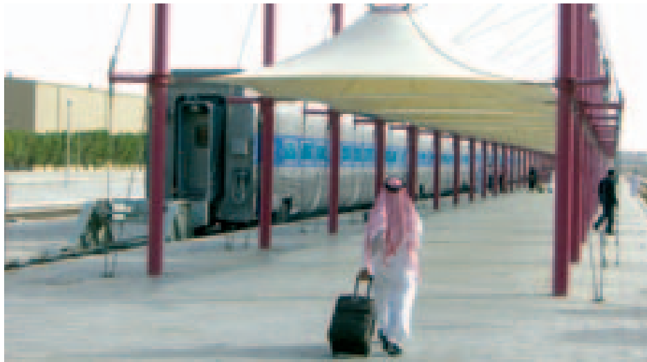
High speed rail links will cut travelling times between Makkah, Madinah and Jeddah.
